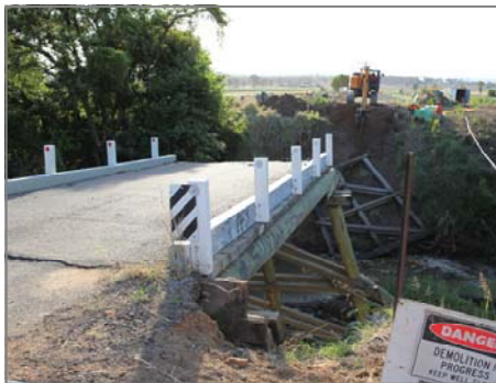
Above: removal of the damaged bridge
