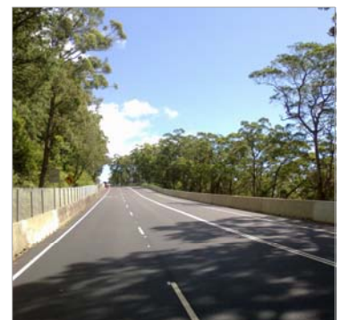
Above: Completed works at Fig Trees, Cunningham Highway.
