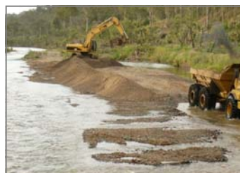
Above: Restoration works underway at Savages Crossing
