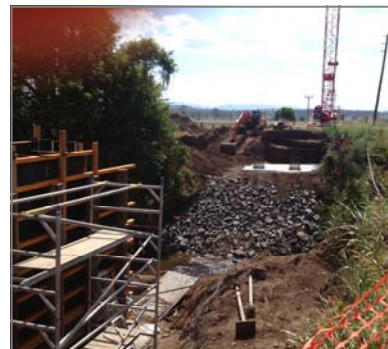
Above: construction of headwall and piles at abutments.
