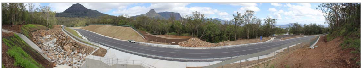
Above: Claytons Gully section of the Cunningham Highway, Cunninghams Gap, after the completion of works in December 2012.
