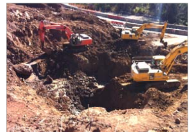
Above: Earthworks at Claytons Gully
