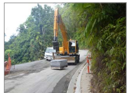
Below: restoration work on Lake Morris Road
