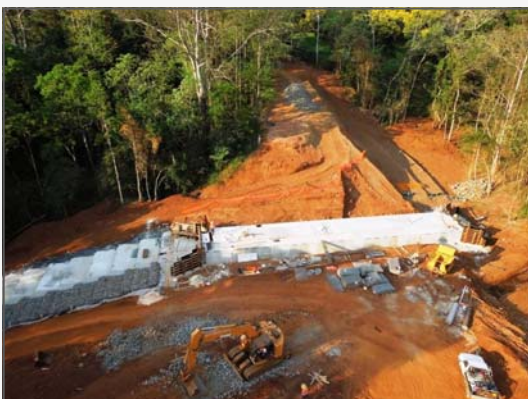
Above: Esk-Hampton Road culvert replacement in progress in October 2012
