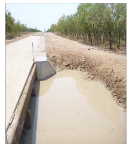
Above: completed works on another section of Floraville Road.
