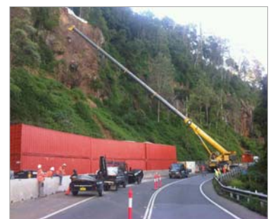
Above: Gravel filled shipping containers at Gap Creek, Cunningham Highway.
