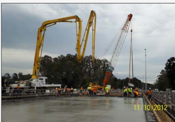
Above: AJ Wyllie Bridge pouring first span, 11 October 2012
