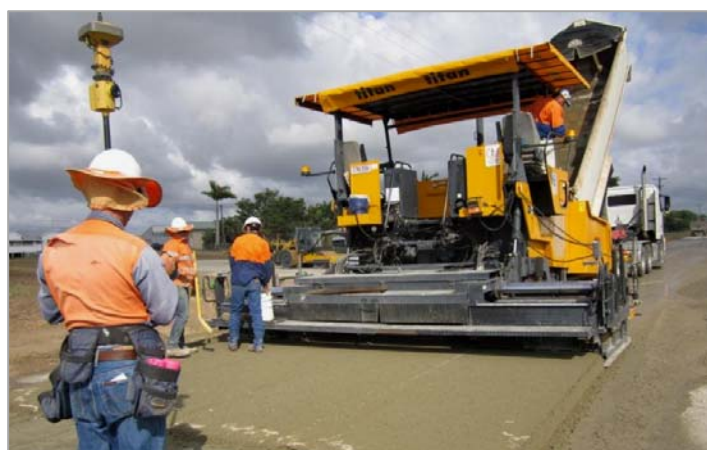
Above: Bruce Highway (10G) paving of cement modified base.
