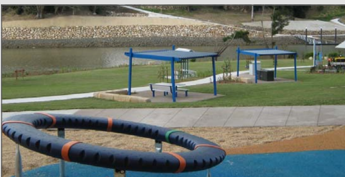
Above: New park facilities - The new children's playground and climbing wall have been situated to improve its flood immunity
