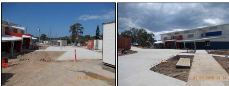
Above: Progress of completion of Cyclone Shelter - Yeppoon SHS
