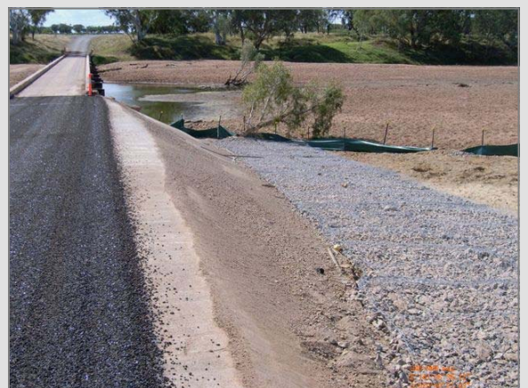
Above: a completed project and the environment left unharmed
