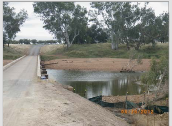
Above: fencing off the trees within the construction zone
