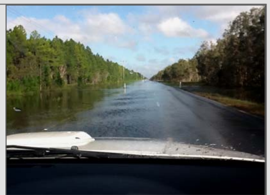
Right: 2012 Natural disaster Flooded on 6 March 2012 after reconstruction works partially completed
