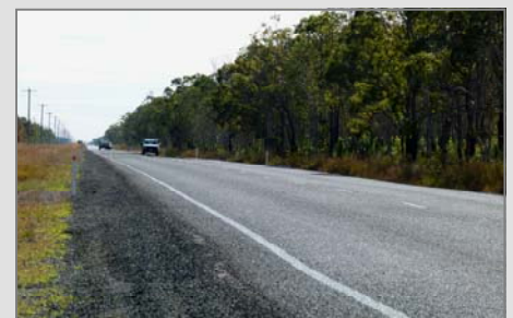
Above and below: July 2012 - Pavement stable after flooding and traffic usage on 5 July 2012
