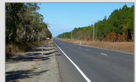
Above and below: July 2012 - Pavement stable after flooding and traffic usage on 5 July 2012
