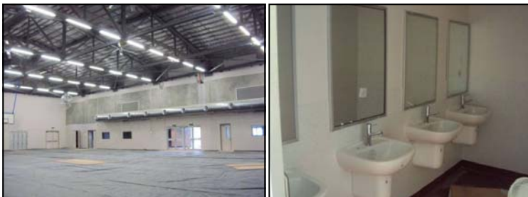
Above: Progress of completion of Cyclone Shelter - Bowen SHS
