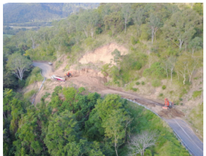
Above: Sarina Range – preliminary works at landslide site
