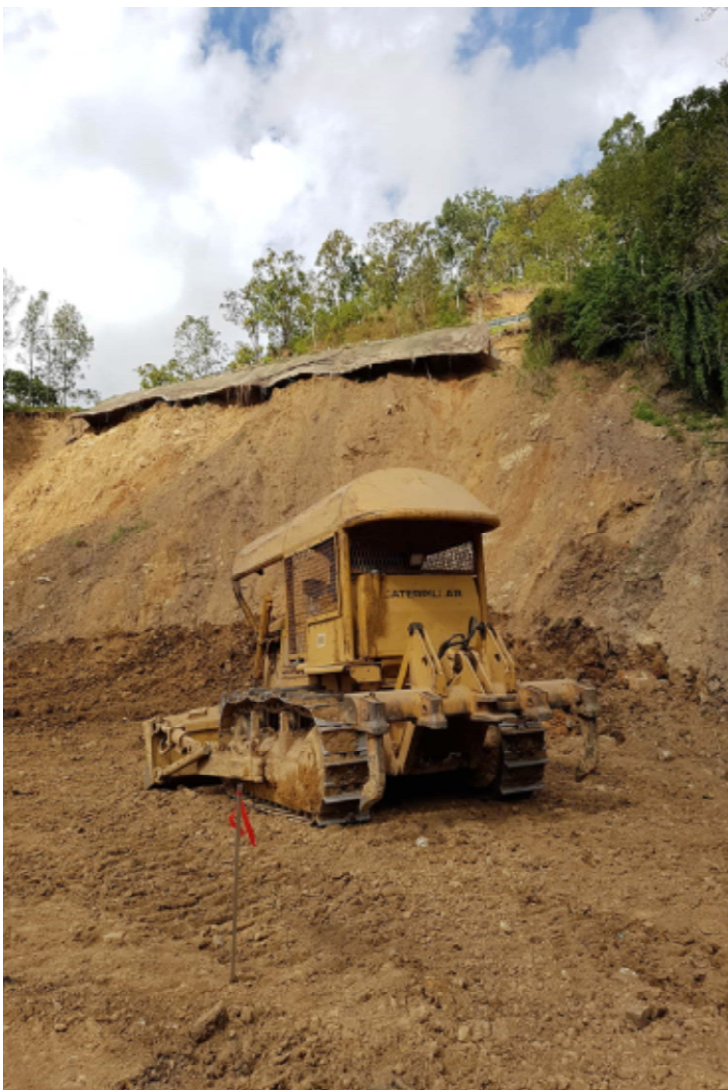
Above: Sarina Range – preliminary works at landslide site
