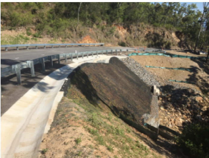
Above: Pilbeam Drive in Rockhampton Regional Council after Betterment completion works
