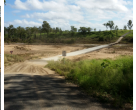
Betterment works following impacts of Severe Tropical Cyclone Debbie
