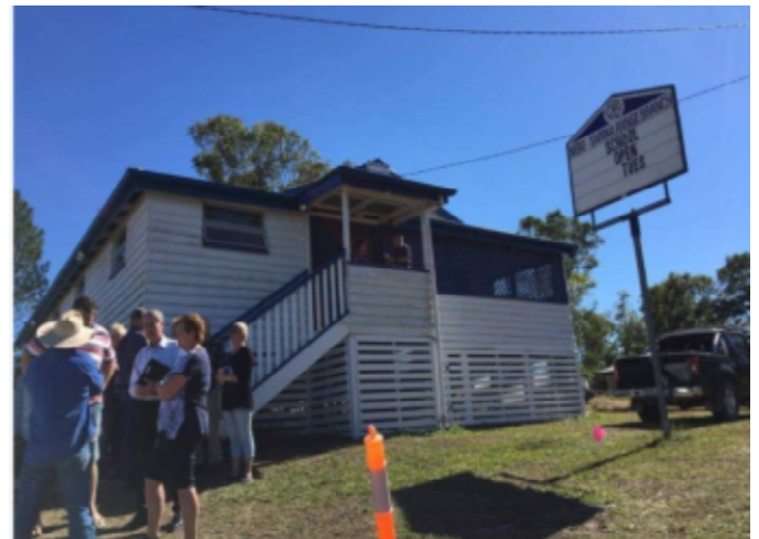
Above: Swayneville State School temporary campus site at Colston Park
