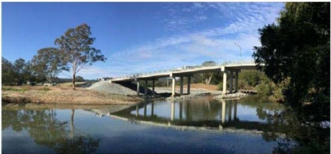
The completed Alan Wilke Bridge project
