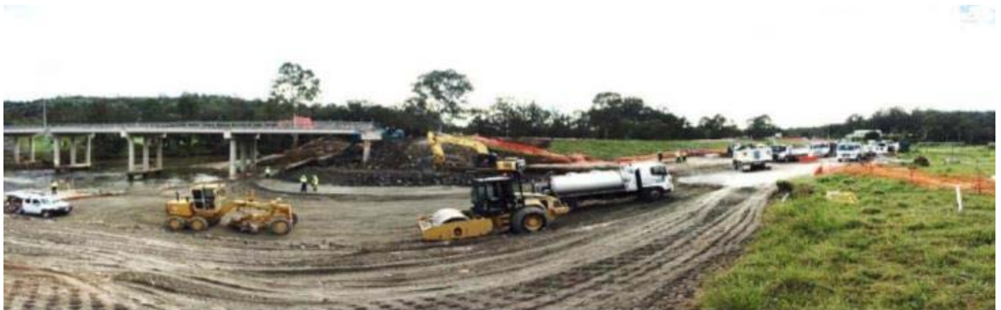
Works on site at the Alana Wilke Bridge – 30 June 2017
