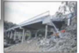
The Alan Wilke Bridge has reopened after four months.
