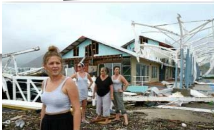
IDIST: Shute Harbour suffered significant damage as a result of Cyclone Debbie.
