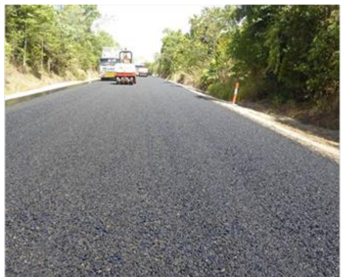
Above: El Arish–Mission Beach Road – pavement reconstruction
