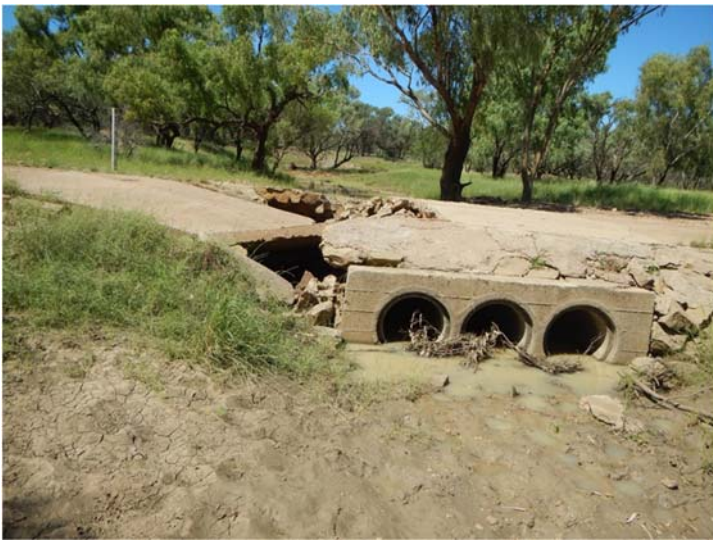
One of Longreach Regional Council's 2014 event restoration projects - damage to Yaraka River Road floodway at Isisford (left) and following restoration works (right)
