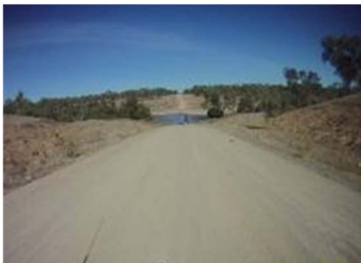
Burke Developmental Road following completion of reconstruction works
