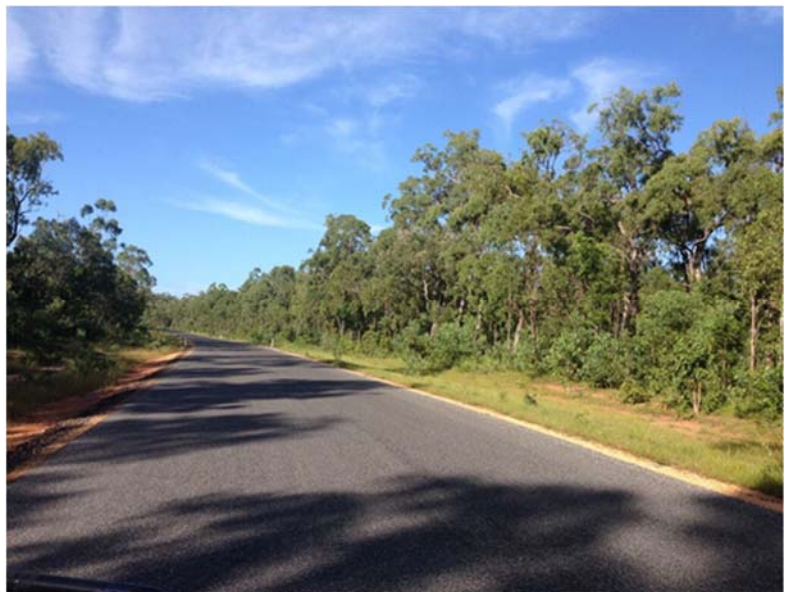
The upgraded Weipa-Mapoon Road is now stronger and more resilient to future damage.
