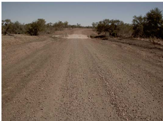
Gregory Downs–Camooweal Road following completion of reconstruction works
