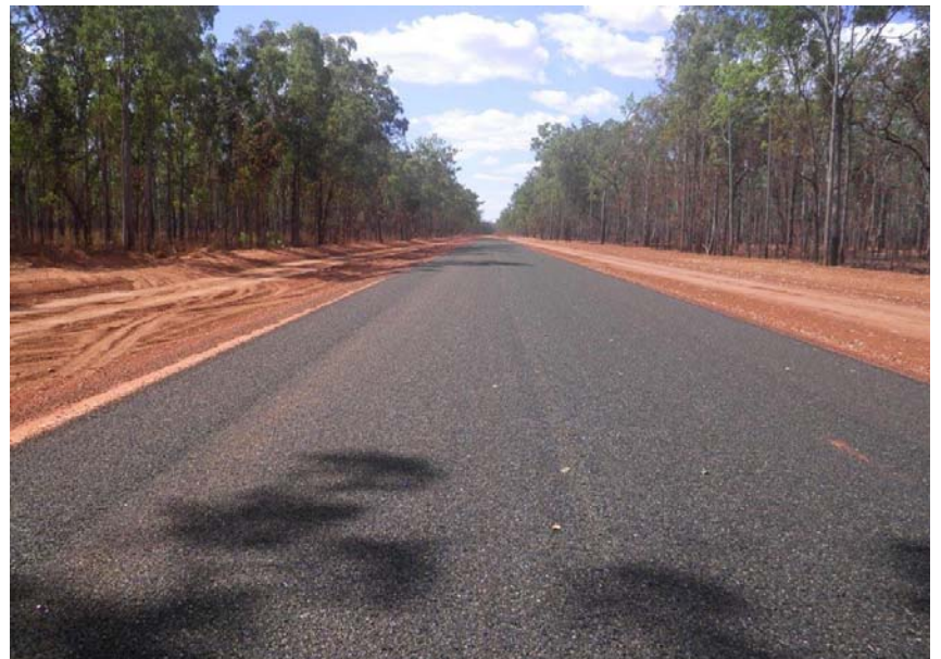
Aurukun Access Road – unsealed sections showing deep scouring damage (left); and with improved resilience to flooding following bitumen sealing (above)
