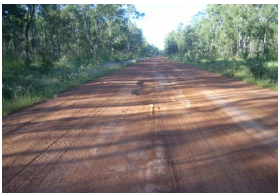
Aurukun Access Road – unsealed sections showing deep scouring damage (left); and with improved resilience to flooding following bitumen sealing (above)
