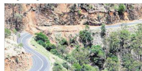
A landslide on the Burnett Hwy on the Mount Morgan range. PHOTO: ALLAN REINIKKA ROK10213AFLOODAB
