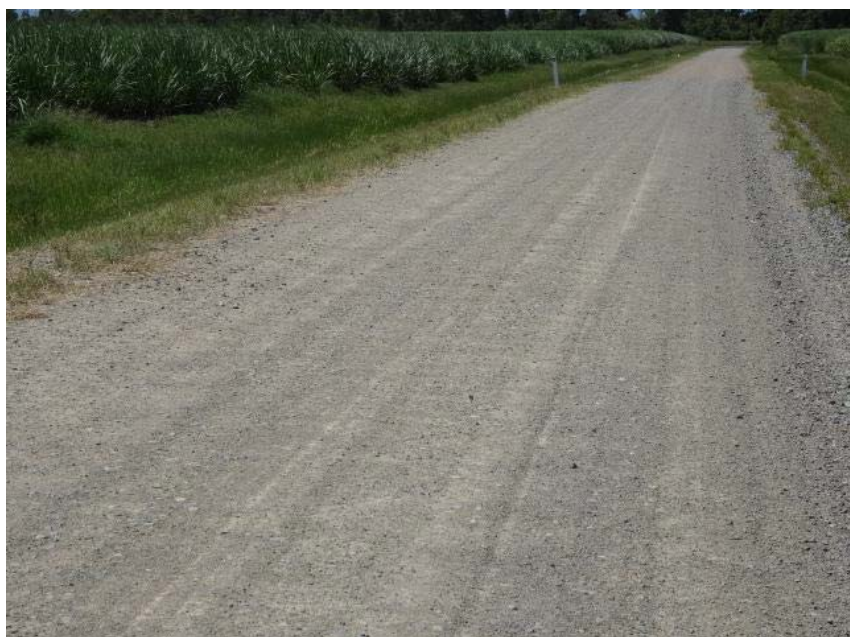
Right: Old Cardwell Road - following completion of reconstruction works
