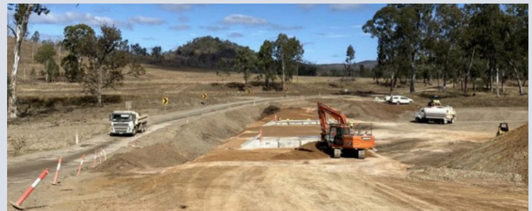
Image: Gladstone–Monto Road – road excavation on south side
