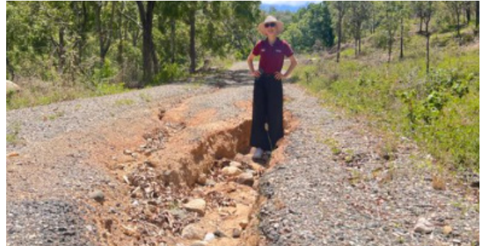
Get Ready Queensland on an asset inspection on Palm Island
