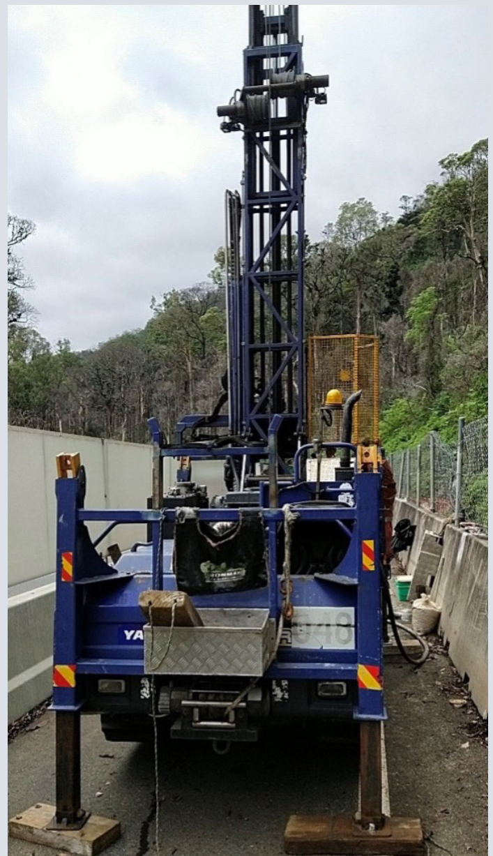
Cunninghams Gap – onsite geotechnical investigations
