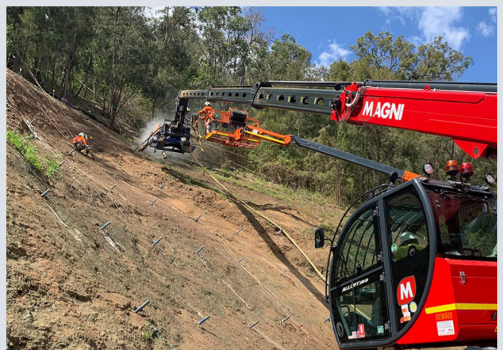
Lamington National Park Road – soil nailing in progress (September 2022)
