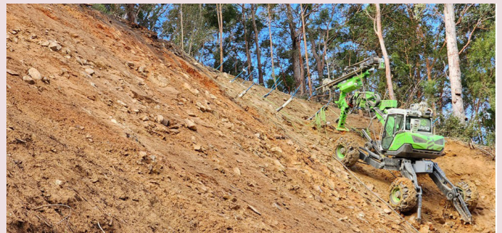
Gold Coast–Springbrook Road – spider rig undertaking soil nailing on Site 8 (April 2023)
