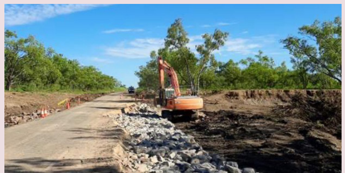
Wills Developmental Road (Julia Creek–Burketown) – installing rock base (April 2023)
