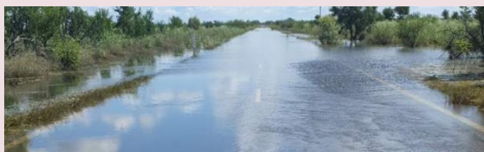
Wills Developmental Road (Julia Creek–Burketown) – extensive areas underwater as a result of Northern and Central Queensland Monsoon and Flooding (March 2023)
