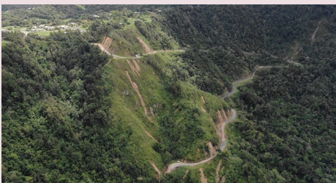
Mackay–Eungella Road – multiple landslips caused by Northern and Central Queensland Monsoon and Flooding event (January 2023)
