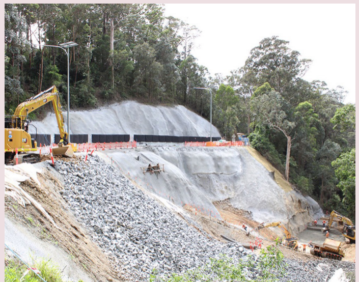
Beechmont Road – works in progress at major embankment failure site (February 2023)
