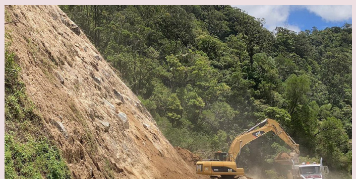
Mackay–Eungella Road – emergency works in progress (January 2023)
