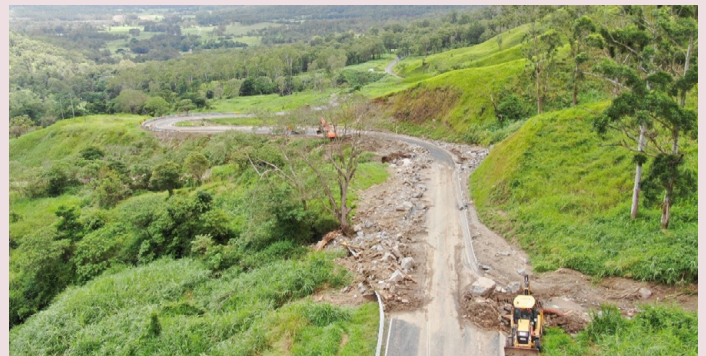
Mackay–Eungella Road – emergency works in progress (January 2023)
