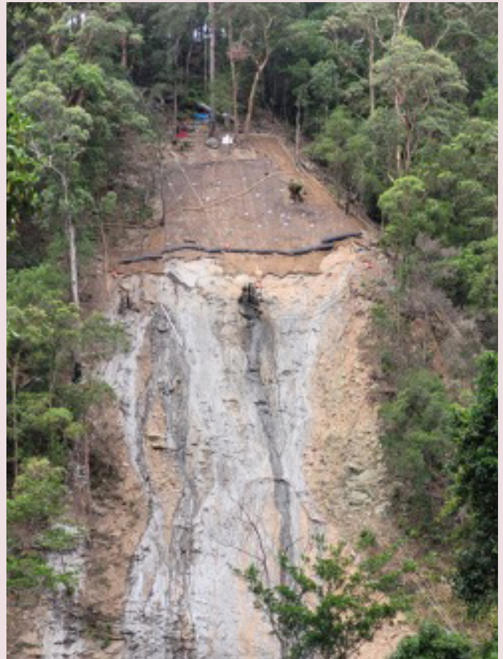
Gold Coast–Springbrook Road – works in progress at main slip site (December 2022)
