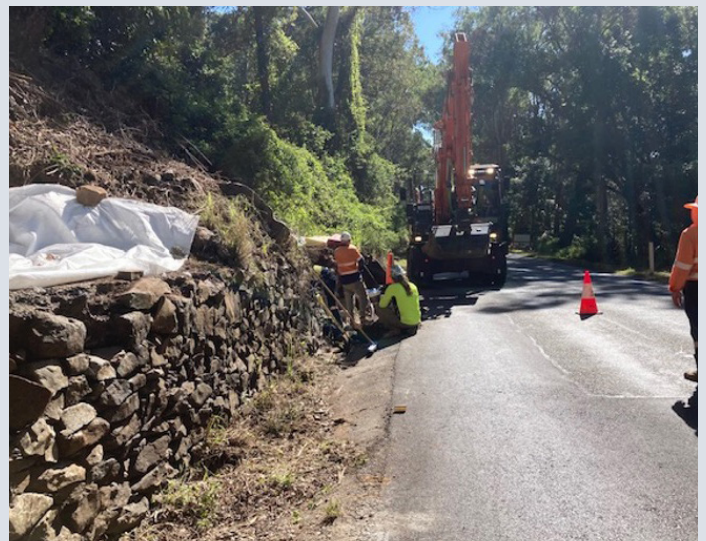
Tamborine Mountain Road – dry-stone wall works in progress
