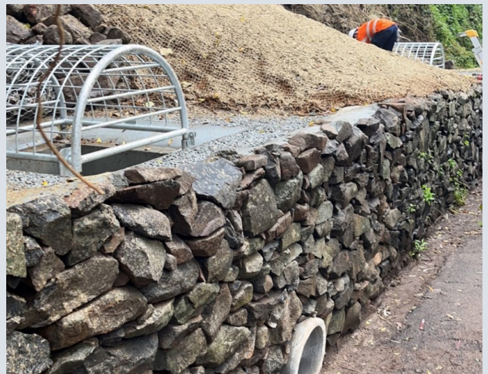
Tamborine Mountain Road – completed works (June 2023)
