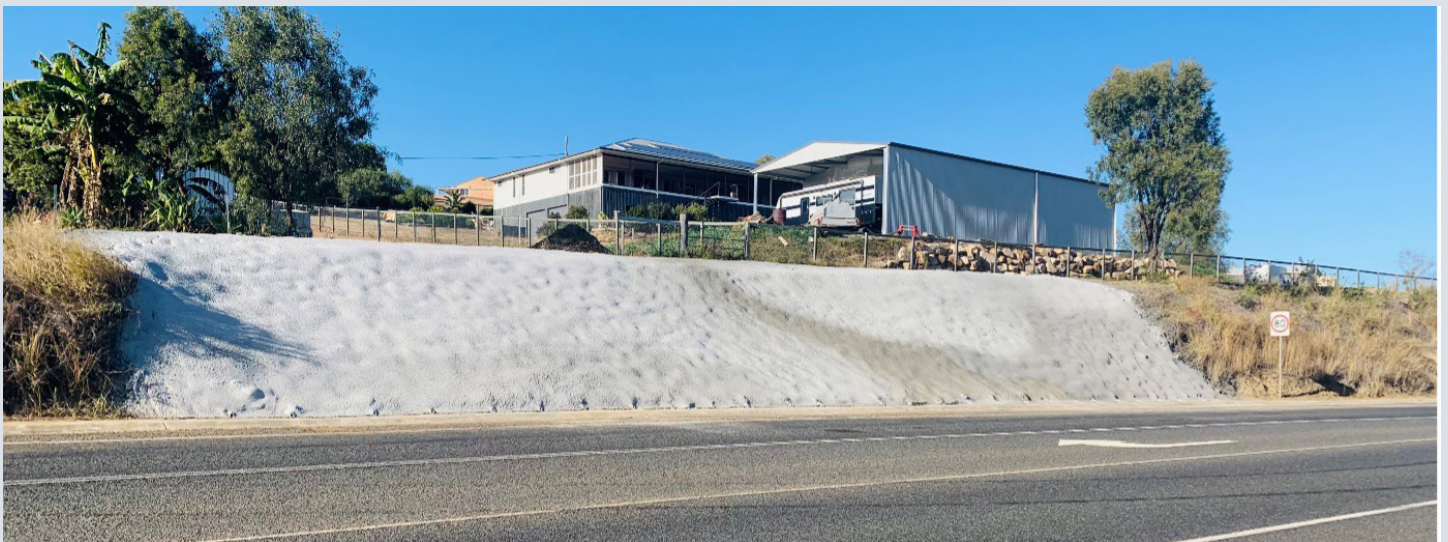
Tamborine Mountain Road – completed works (June 2023)
