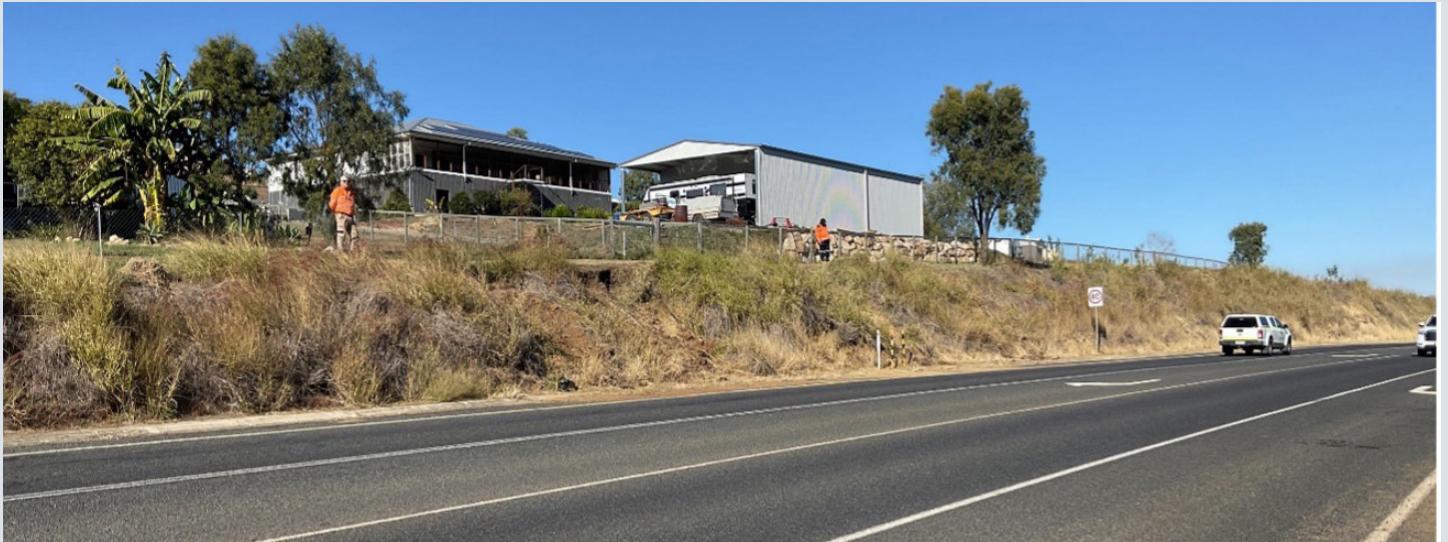
Tamborine Mountain Road – completed works (June 2023)
