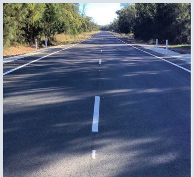
Betterment works complete on the Moonie Highway
